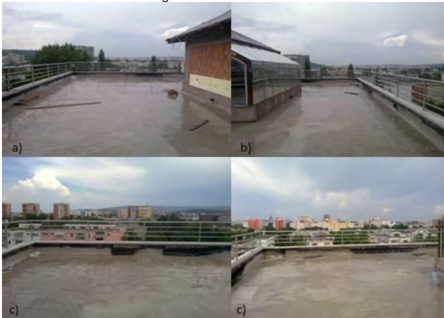
Fig. 2 The roof before rehabilitation
