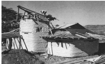
Fig. 9 House built from continue raffia tubes filled with earth, Brazil (World Heritage, 2012)
